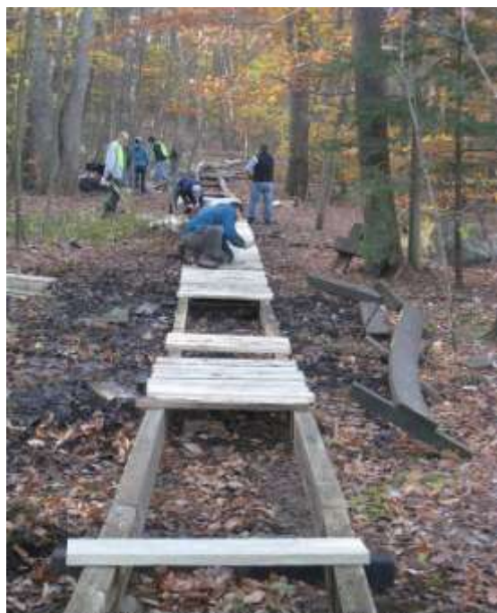
Paint Mine Boardwalk
